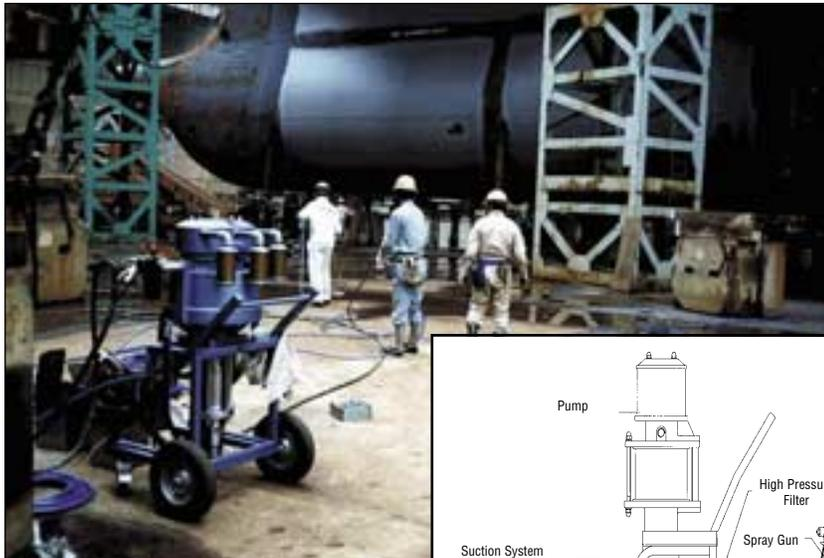
A typical airless spraying operation (above) and a close-up of an airless spray rig (right)
