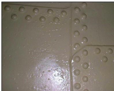
This riveted fuel oil tank was sealed with an elastomeric urethane to prevent leaking.
