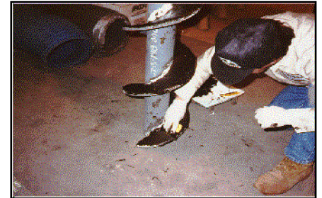
Hand-applied top coat of ARCOR™ S-20
