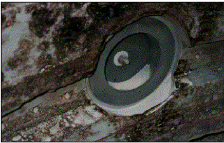
Valve body surface ready for coating
