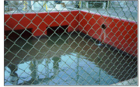
Basin repaired and in service
