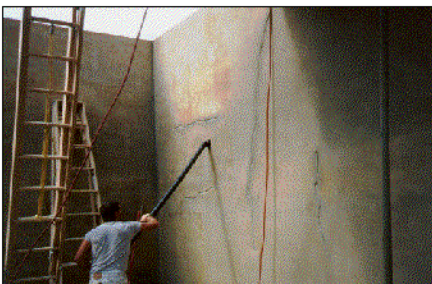
Cleaning cracked wall surface in basin
