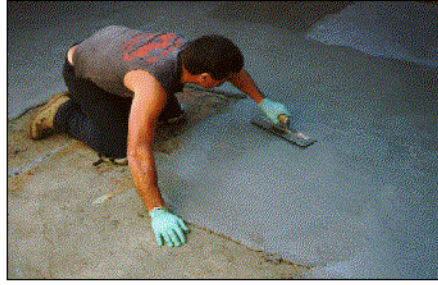
Application of ARCOR™ ARCRETE
