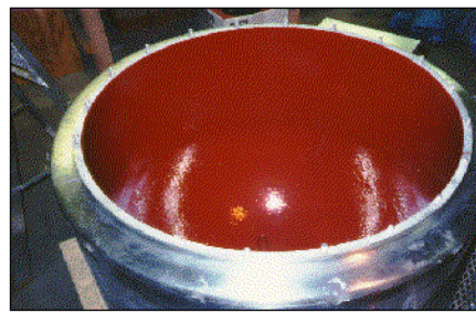
Spray Application of ARCOR™ S-20
