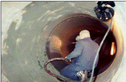
Blasting surface clean
