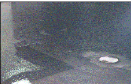
20 mils EE-79 . Area around drain rebuilt
