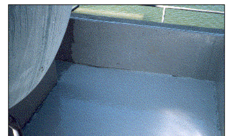
Topcoat with EE-11 for Finished DFT of 40 mils.
