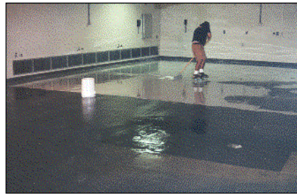
Application of 20 mils ARCORM™ EE-71
