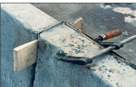
ARCRETE used with Polypropylene Form to Rebuild Damaged Walls
