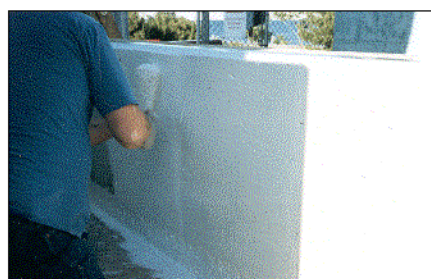
Roller Applied EE-11 Prime coat.
