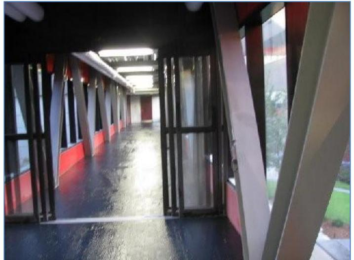
The linear ridges provide channels for movement of water and other liquids, especially in heavy rain. Additionally, they allow for easier cleaning than a more traditional non-skid aggregate scatter.
