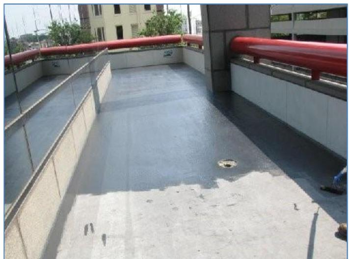
The existing flooring was removed and the concrete was prepared using a scarifier with dust collection. Areas were degreased as needed and diamond grinders were used to remove imperfections and to v-out cracks. Finally, a full clean by power wash.
