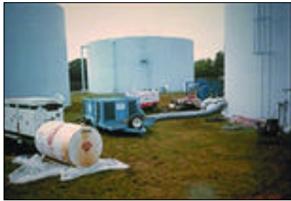
Dehumidification equipment set up for painting operations inside three tanks.
